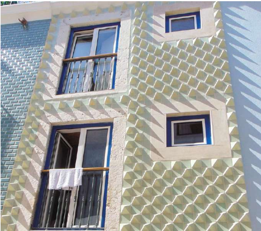
Fig. 09· Lisbon, Friendly Border Apartment, façade, Maria Ana Vasco Costa (b. 1981), 2016
