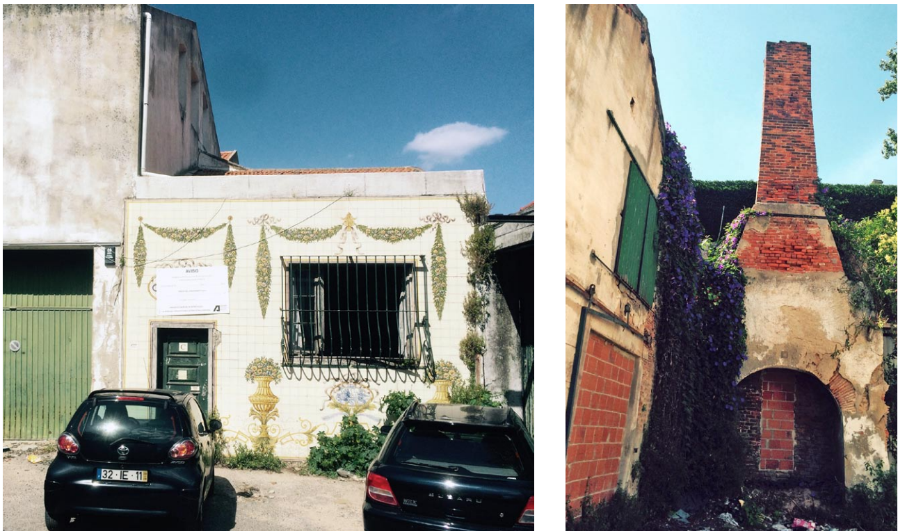
Fig. 01 · Constância Factory, entrance to the shop and exhibition room (right) and old wood firing kiln (left) (photos by Silvia Pereira, June 2017)
