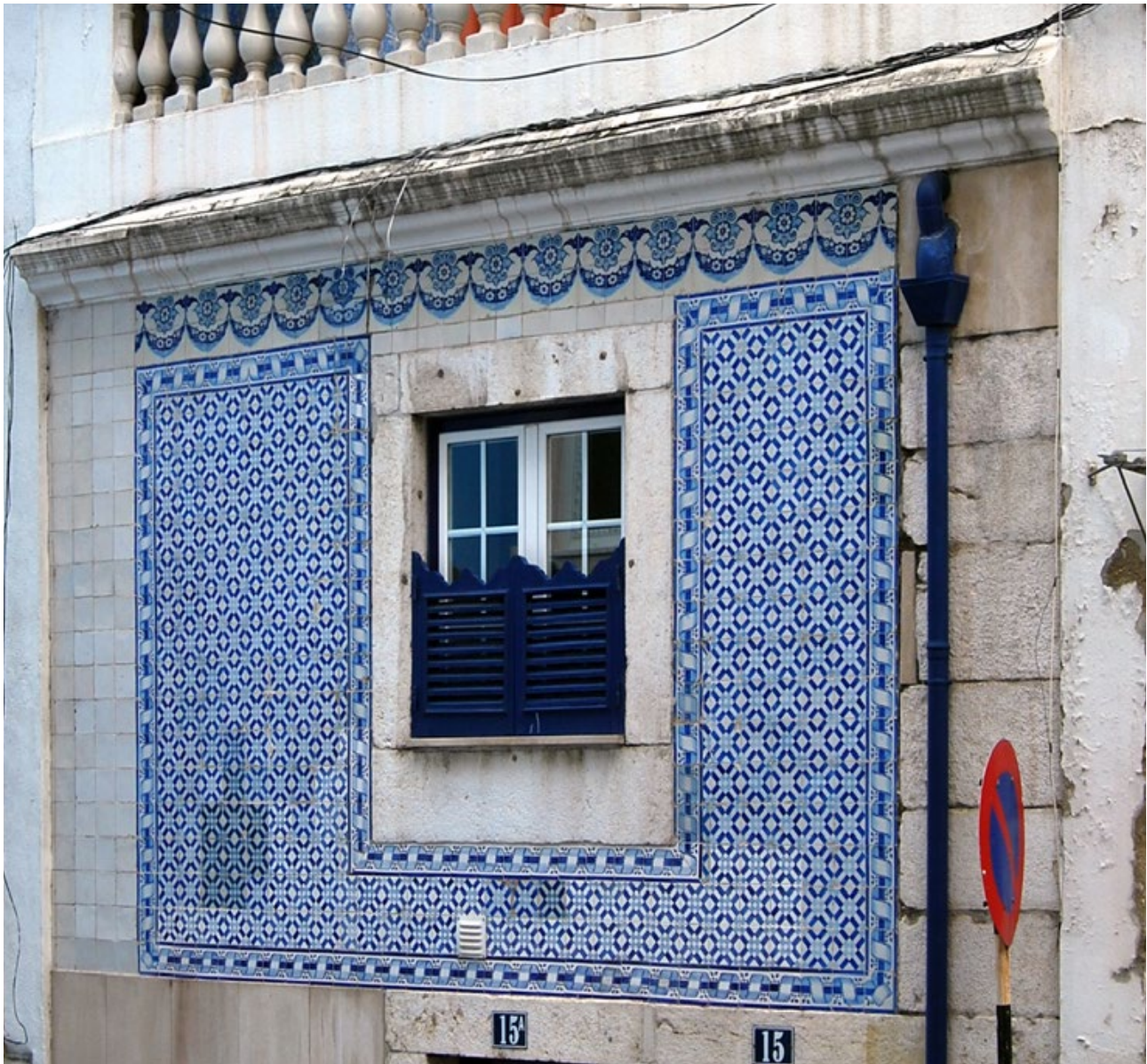
Fig.2 - Early façade lining with azulejos by Fábrica Roseira at Calçada do Cardeal 15. Besides the use of full-sized azulejo frames and double row frieze, all characteristic of the early decades of façade lining in Lisbon, another archaic feature is noteworthy: the left side make-believe stone corner made of white azulejos . Notice that the azulejo pattern is inspired by the checkered “ enxaquetado ” patterns used in Portugal in the 17 th century and seen e.g. in the church of the former Pena Convent in Sintra (photo by Maria de Lurdes Esteves, 2012)
