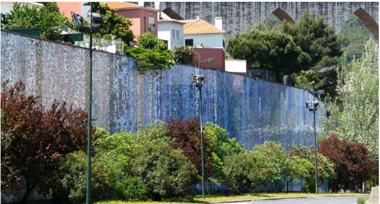
Fig.1 - Embankment wall, 1972-1982, João Abel Manta (1928), Calouste Gulbenkian Avenue, Lisbon (photo by Ana Almeida)
