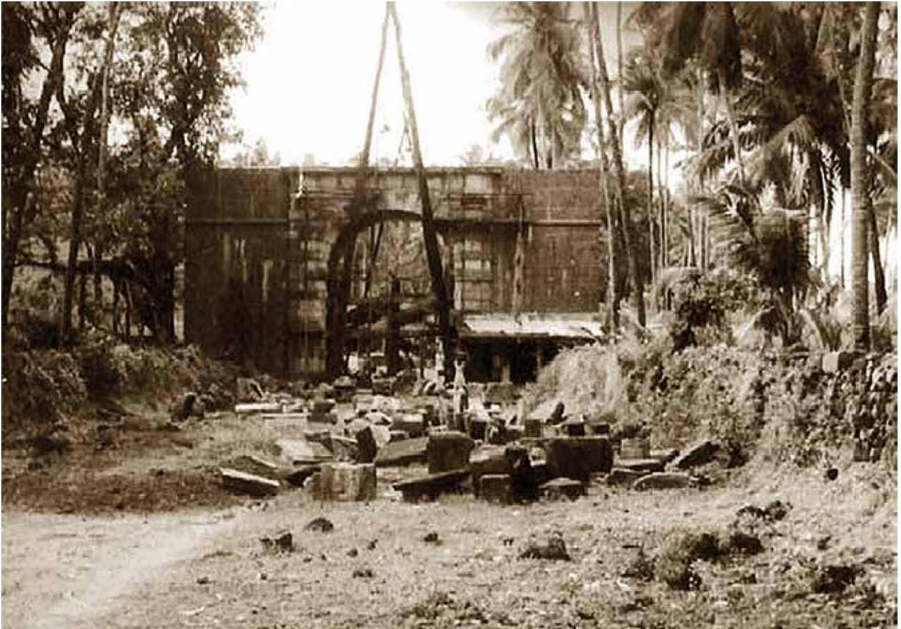
Fig. 06. Arch of the Viceroys in Old Goa, India, during its reconstruction after the collapse as a result of the restoration carried out by Baltazar Castro, 1954 (source: NUNES, Antonieta dos Santos; CRUZ, João Paulo – Um Testemunho de Vida: Capitão Manuel Sidónio dos Santos Nunes . Figueira da Foz: Companhia da Palavra, 2011)
