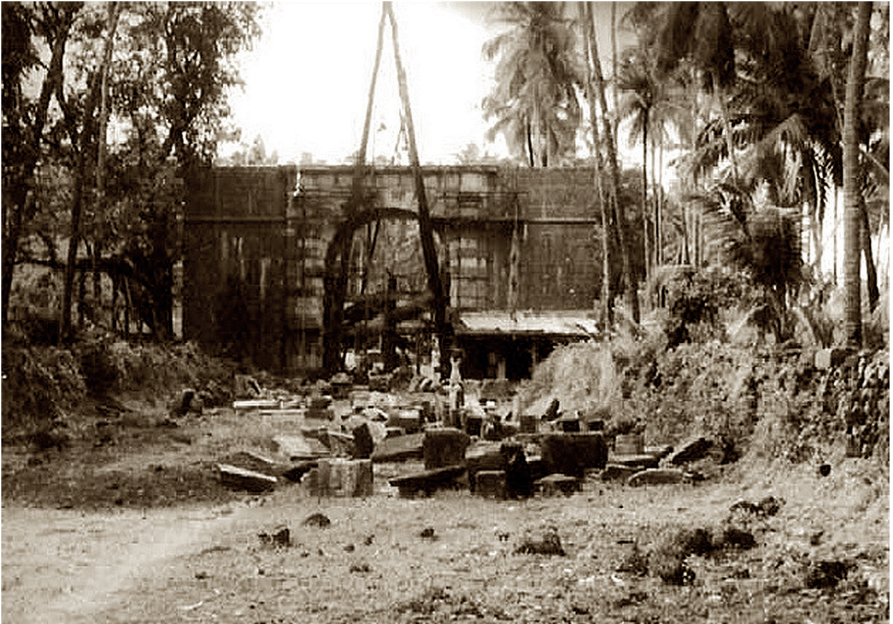
Fig. 06. Arch of the Viceroys in Old Goa, India, during its reconstruction after the collapse as a result of the restoration carried out by Baltazar Castro, 1954 (source: NUNES, Antonieta dos Santos; CRUZ, João Paulo – Um Testemunho de Vida: Capitão Manuel Sidónio dos Santos Nunes . Figueira da Foz: Companhia da Palavra, 2011)
