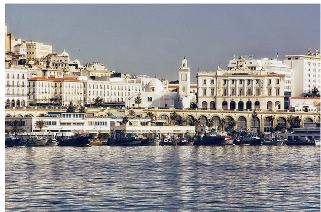
Fig. 08 · The same façade today, heavily modified by the French in the 19 th century (source: Farouk Toumi, 2016).
