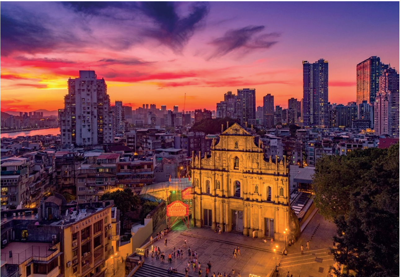
Fig. 11 - Ruins of St Paul's, façade of the old Church of Mater Dei (source: Chan Hin lo, 2016)
