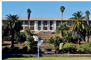
Fig. 19. Government Office Building in Windhoek, Namibia, by Gottlieb Redecker, 1912-13 (source: Wikipedia, photo by Zairon)
